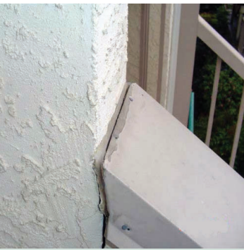
Lack of adhesion between sealant, flashing and stucco will allow water ingress at this building detail (balcony connection).
