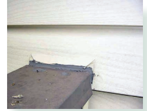
The sealant at the guardwall connection to wall has begun to fail; a regular inspection and maintenance plan will detect this type of failure before it converts into a costly repair item.
