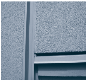
Sealants found at exterior cladding joints require maintenance to ensure adequate building envelope performance.
